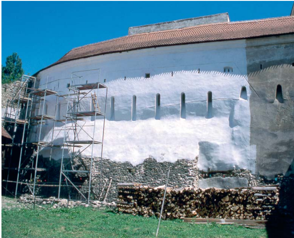
New render and paintwork on the curtain wall in Prejmer/Tartlau
