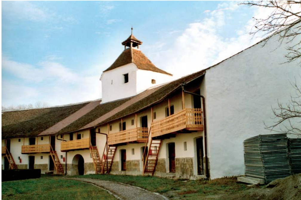
Staircases and banisters in front of the escape chambers and pantries in Harman/Honigberg had to be replaced with authentic replica. Linden tree soaked in linseed oil was used.
