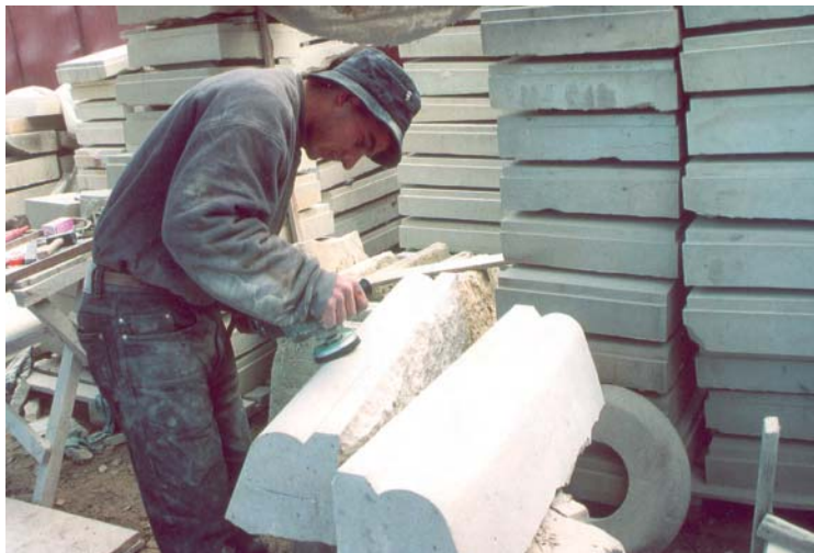
Cutting of stones from Sânzieni (Harghita district) for the church's foundations
