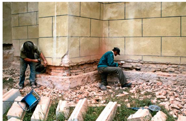
The weathered foundations were removed in the spring of 2004 and replaced with new stones
