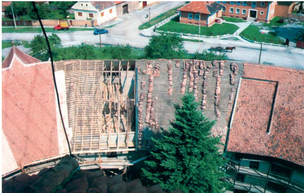
Over 600000 special roof tiles (single lap tiles) were used during the renovation of the roof above the outer curtain, which is 800m long and 5m wide at the base
